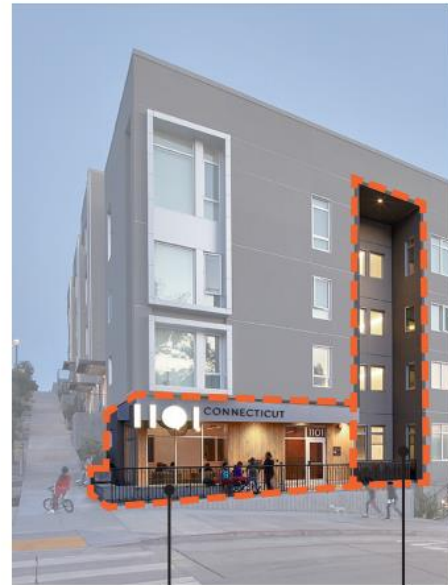
Articulated building corner with public plaza
